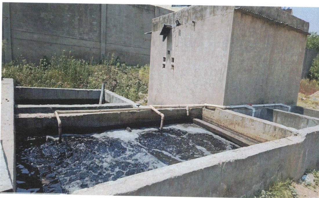
26 KLD LTP WITH NEW LANDFILL SITE
